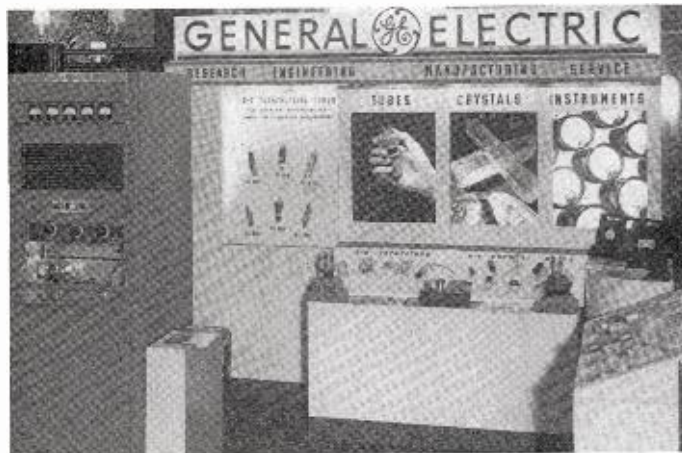
THAT STREAMLINED contraption on the left is not a new General Electric refrigerator, but the new 250-watt FM broadcast transmitter manufactured by GE. It was exhibited at the recent convention of the Institute of Radio Engineers in Boston, along with other GE broadcast innovations and proved to be the only transmitter on display.
